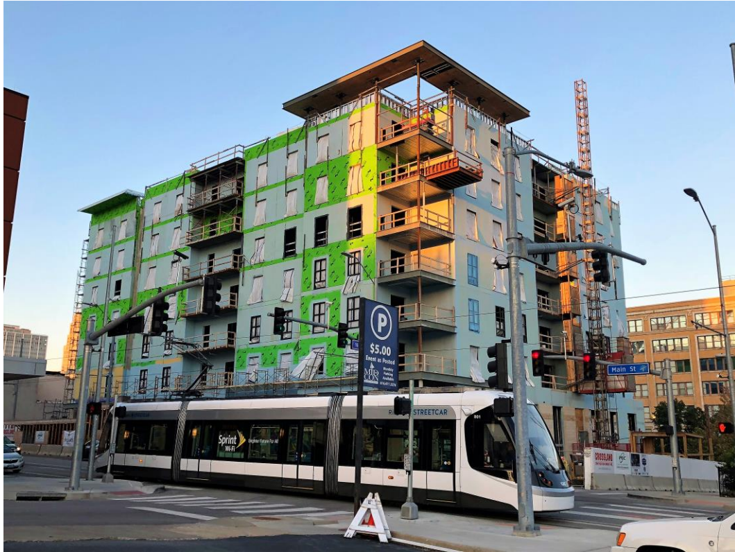
KC Streetcar- Starter-Line - new hotel under construction
