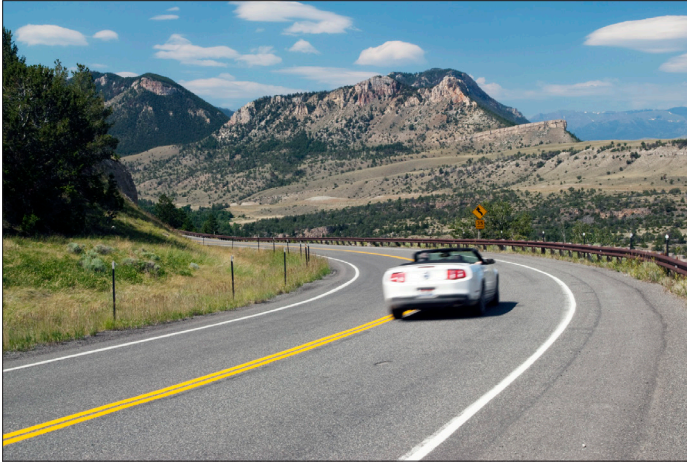
Wyoming's Beartooth Highway Reconstruction Project was included in TIGER I and received $6 million in funding.
